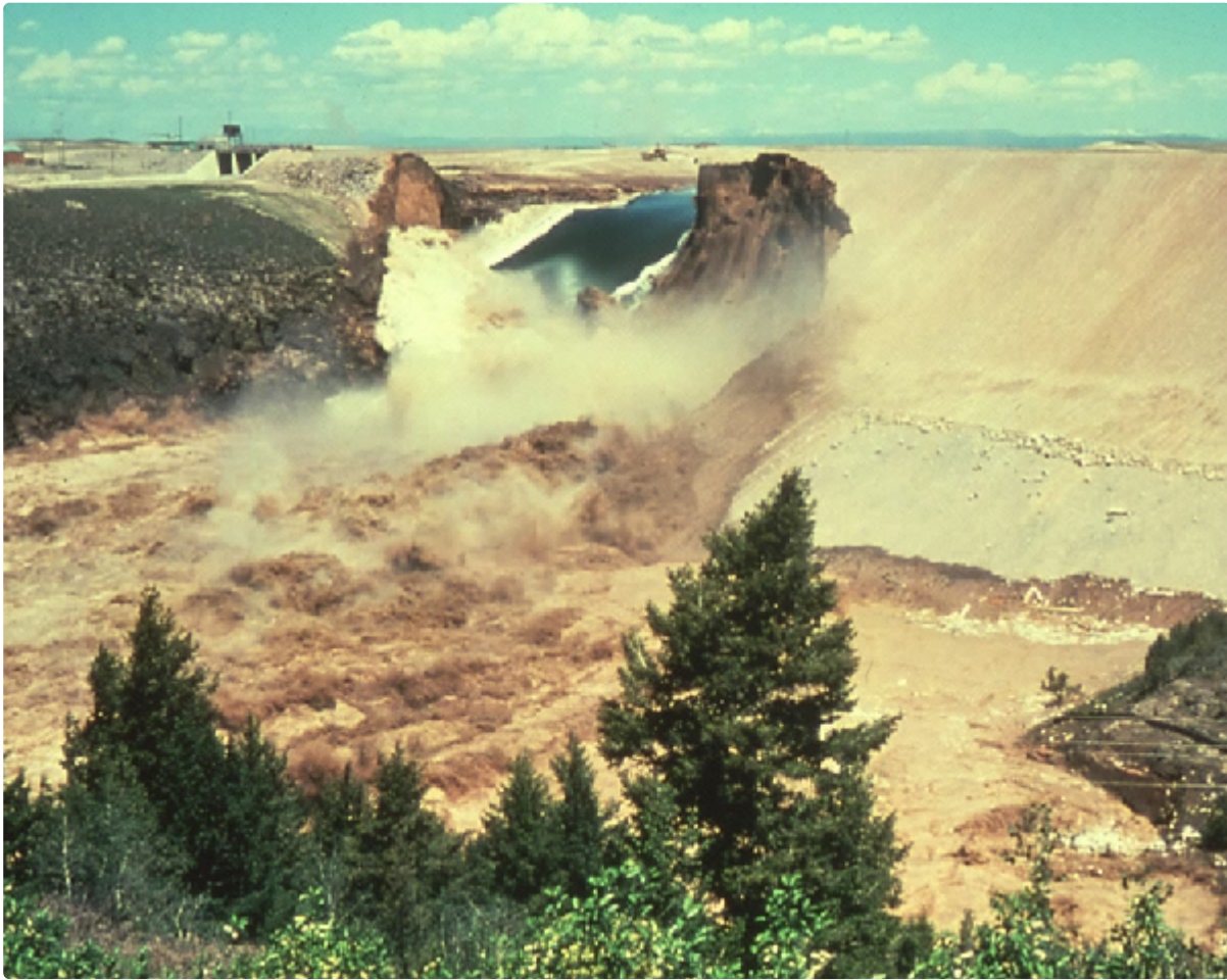
Significant Turbulence and Sediment load during the Teton Dam Failure
